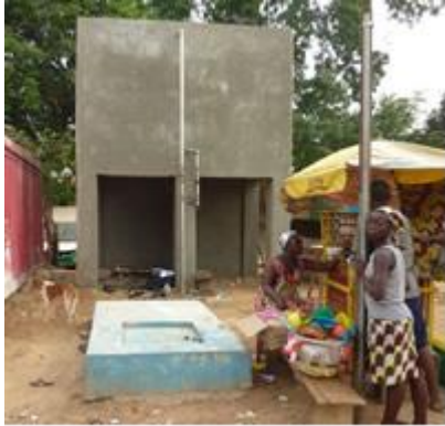
Water tank in Bo market
