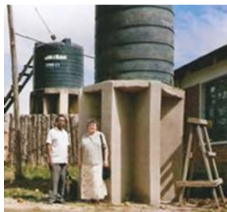
Some Water tanks installed (Tanzania)
